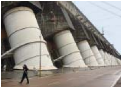
Close-up of the pressure pipelines feeding water into the turbines.
