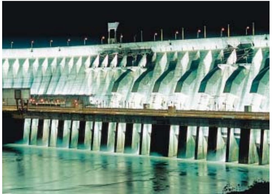
Close-up of the pressure pipelines feeding water into the turbines.
