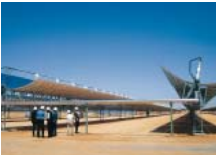
Huge parabolic mirrors dominate the scene at solar thermal power plants.
